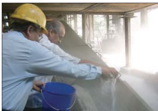
Mixing of plastics waste with stone
