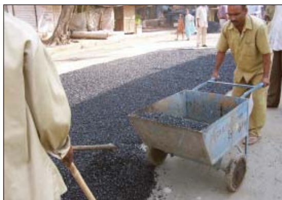
Tar Road laying in progress
