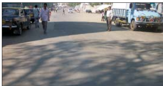
Completed road after 7 days
