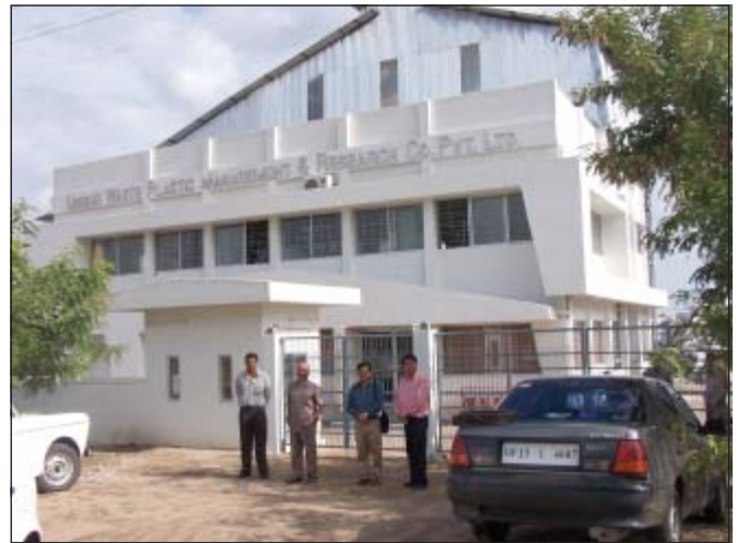
Nagpur Factory which manufactures Fuel from Plastics Waste.
