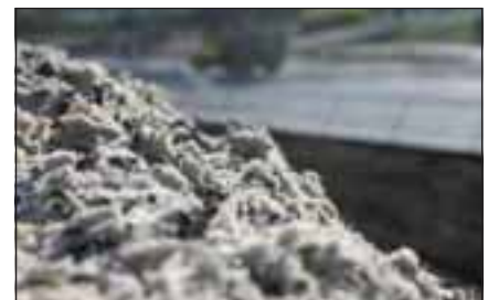
Polytrack consists of using a "cushioning" top layer and sub layers to provide the foundation and vertical drainage pipes.
