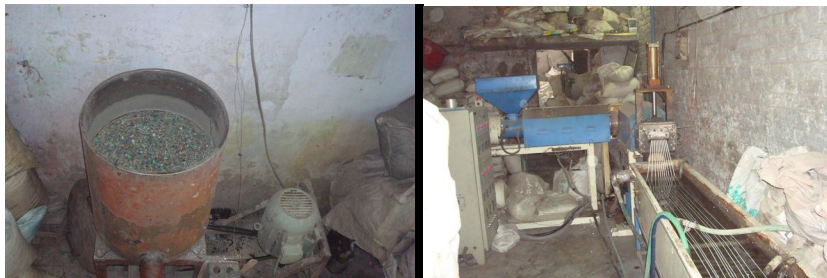
Inadequate Safety measures
