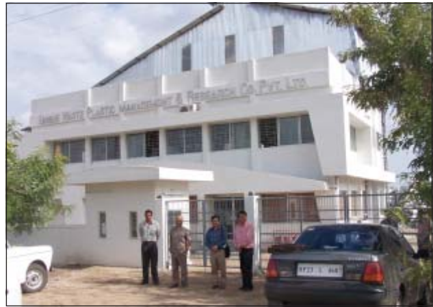
Nagpur Factory which manufactures Fuel from Plastics Waste.
