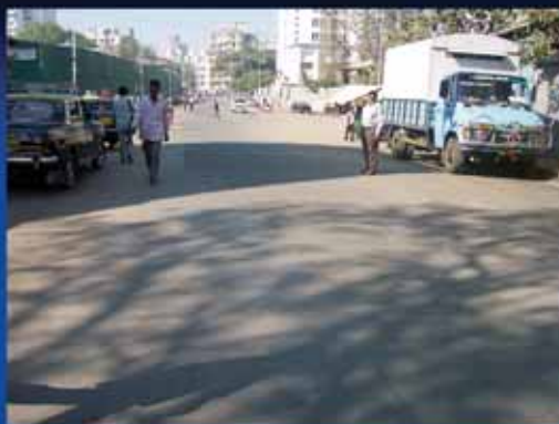
Completed road after 7 days- Mumbai
