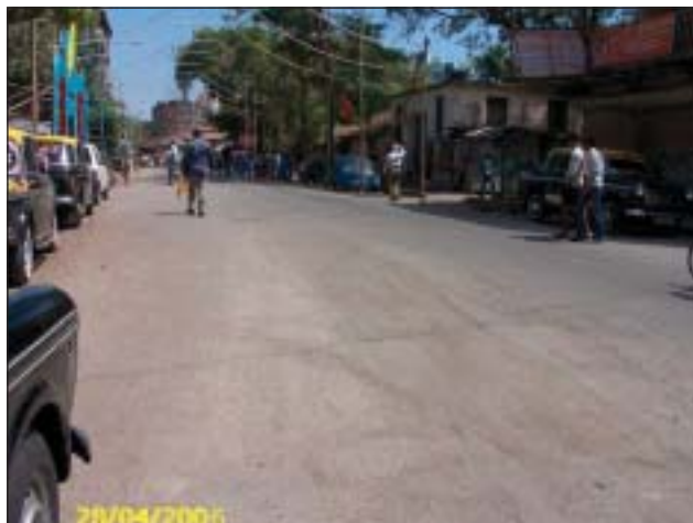
View of the road – 15 months after completion
