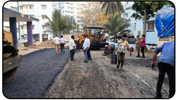
Bituminous Road with Plastics Waste being constructed at Navy Nagar Township, Colaba, Mumbai
