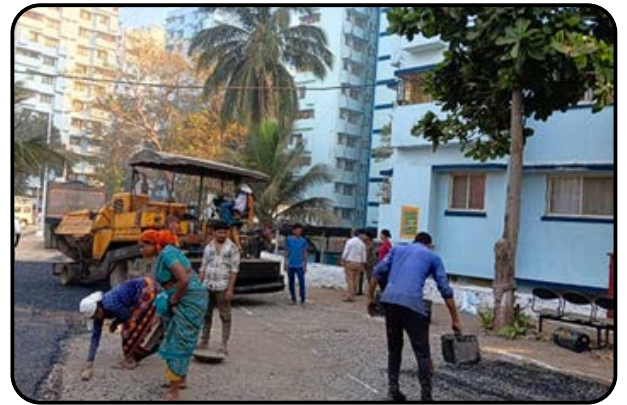
Bituminous Road with Plastics Waste being constructed at Navy Nagar Township, Colaba, Mumbai
